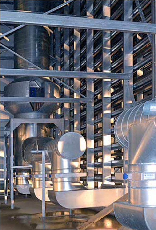
Air circulation systems create the right conditions for constant temperature and humidity distribution inside the curing chamber. Optional: with active temperature and humidity control.
