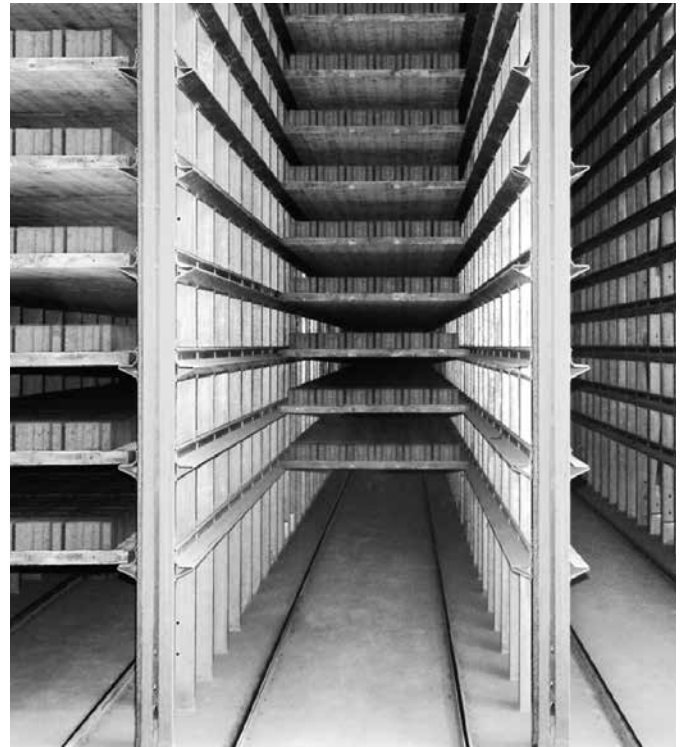
The result is exactly level and height true installation.
