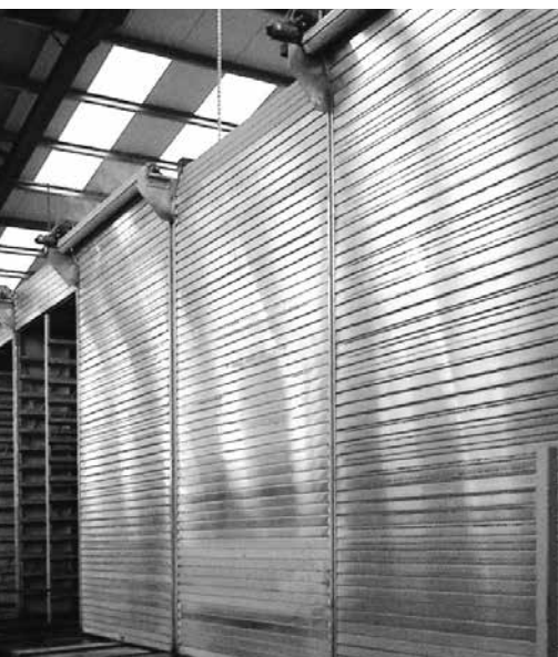
Curing chambers with roller shutters is possible anytime.
